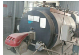
■ Air supply fan for boiler
